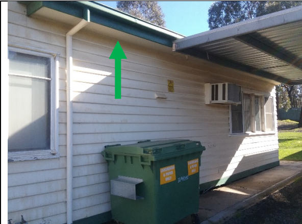
Photo 2: No asbestos detected in sample 1-270721. Cement sheet eaves of House.
