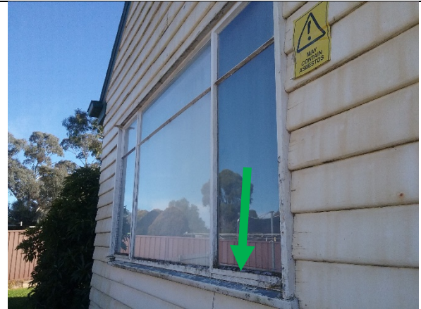
Photo 3: No asbestos detected in sample 2-270721. Window putty of House.
