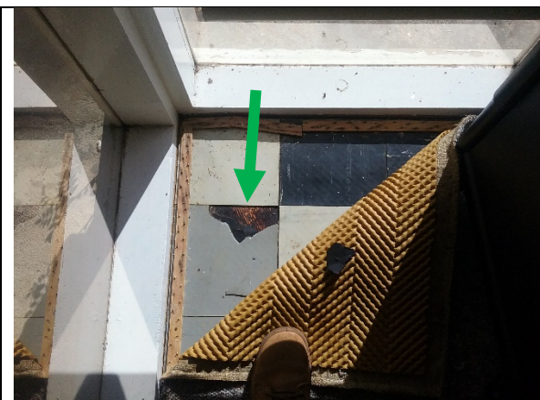
Photo 6: No asbestos detected in sample 5-270721. Vinyl tile beneath carpet floor of Kitchen/Dining.
