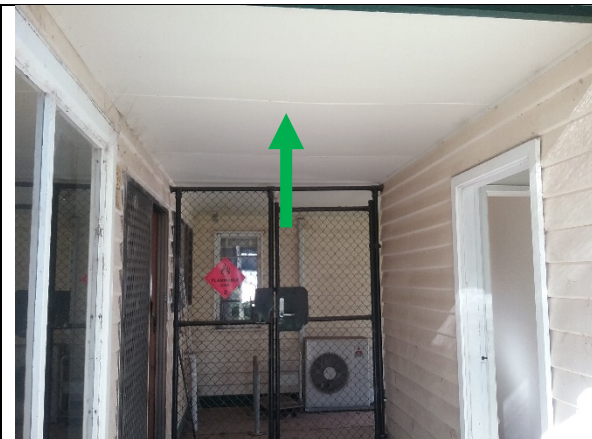
Photo 4: No asbestos detected in sample 3-270721. Cement sheet ceiling of Verandah.
