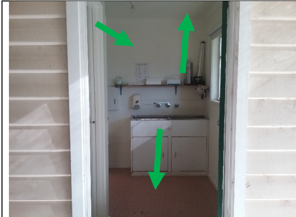
Photo 8: No asbestos detected in sample 7-270721, 8-270721 & 9-270721. Cement sheet ceiling & walls and vinyl sheet floor of Laundry/Toilet.
