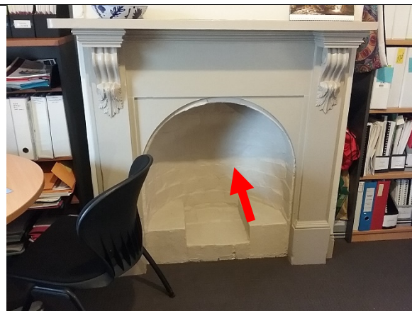
Photo 2: No access inside office fireplace at the time of the audit. Assume asbestos is present until determined otherwise.
