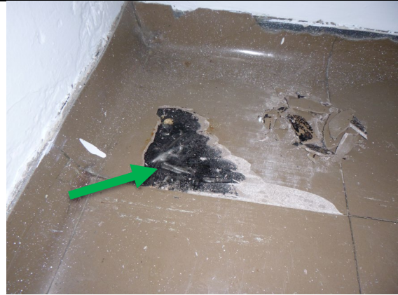
Photo 350: No asbestos detected in sample 2-230721. Black adhesive beneath vinyl tiles in staff toilet.
